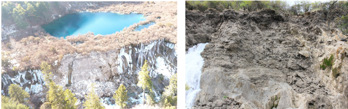
图2 地震后诺日朗瀑布大坝(左:全景,右:局部) Fig. 2 Nuorilang waterfall dam after the earthquake (left. panoramic, right. partial)
