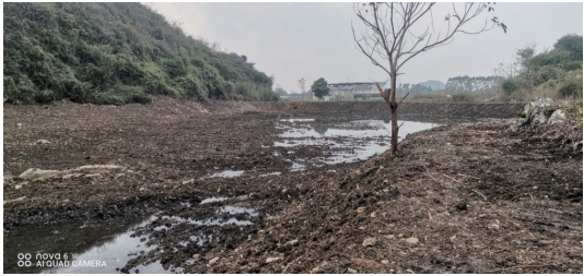
照片 4 清淤后的狮子潭 Photo 4 Shizi lake after the silt clearing
