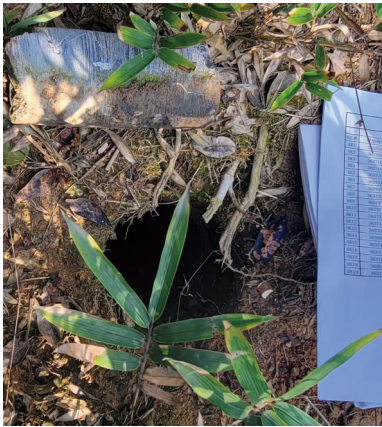
图 16 钻孔岩溶揭露 Fig. 16 Karst exposure of boreholes
