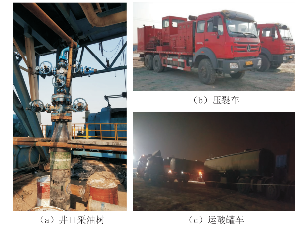
图 4 酸化洗井作业主要设备 Fig.4 Main equipment for acidizing operation
