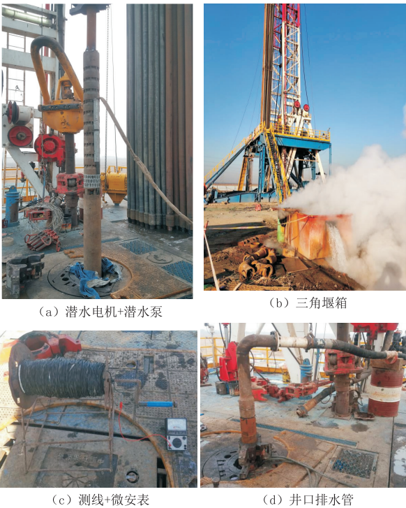
图 5 抽水试验设备 Fig.5 Pumping test equipment
