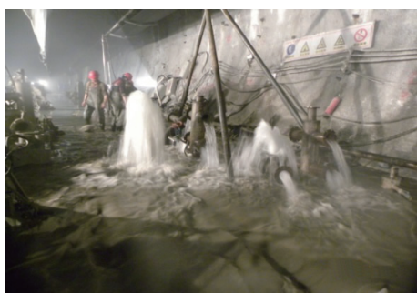
图 7 现场分流减压孔钻孔 Fig.7 Drilling of diversion holes for pressure relief
