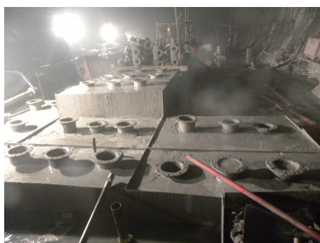
图 6 注浆孔口管预埋及砼浇筑后的沉箱效果 Fig.6 Caisson with the pre-embedded grouting pipe and cast concrete
