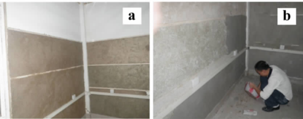
图3 石膏基保温砂浆的施工(a.保温层的施工;b.抹面层的施工) Fig. 3 Construction of gypsum-based thermal insulation mortar (a. construction of thermal insulation layer; b. construction of plastering layer)
