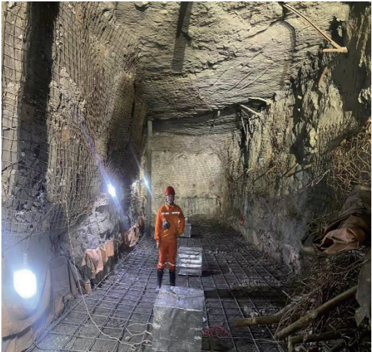
图 6 浮箱式点柱在实验采场安装实景 Fig. 6 Realistic picture of buoyant box point column in test stope
