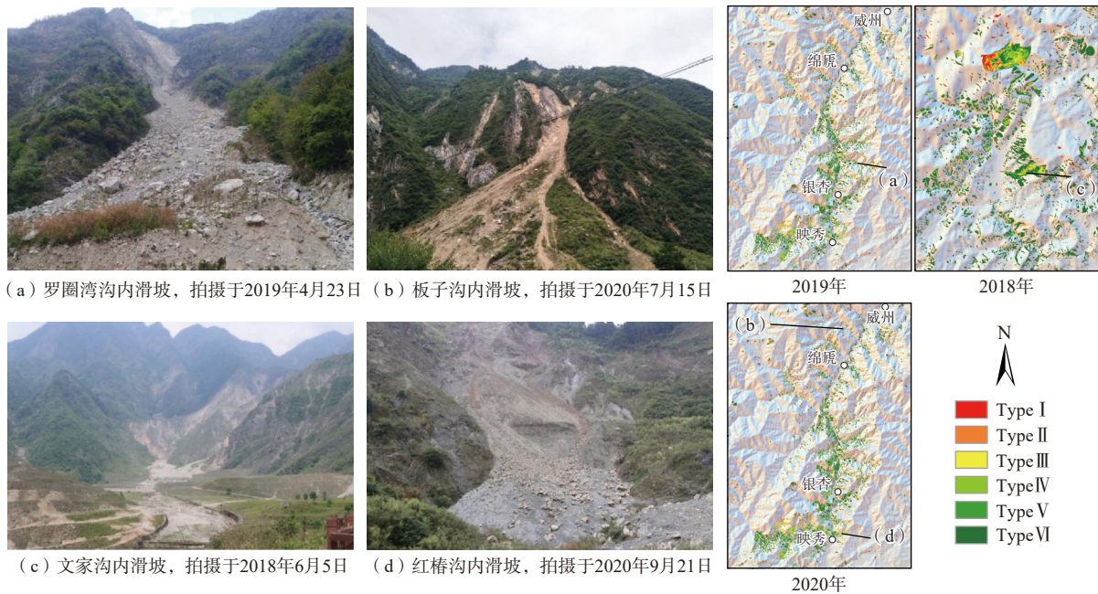
Fig. 11 Landslide materials continuing to transfer downstream from giant landslides
