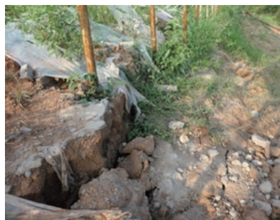
Fig. 3 Surface cracks in the tunnel portal section
