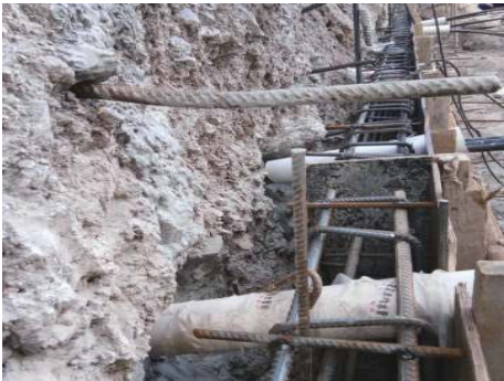
(a) 钢筋笼和预留锚索孔
