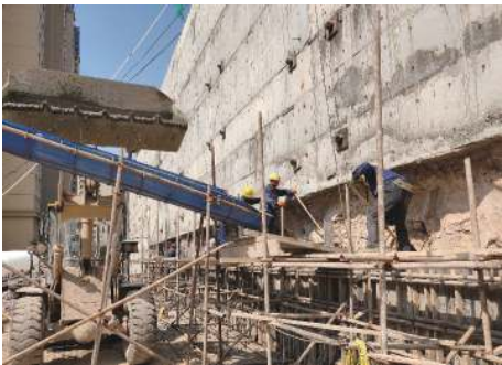
(b) 桩前挂板砼浇注
