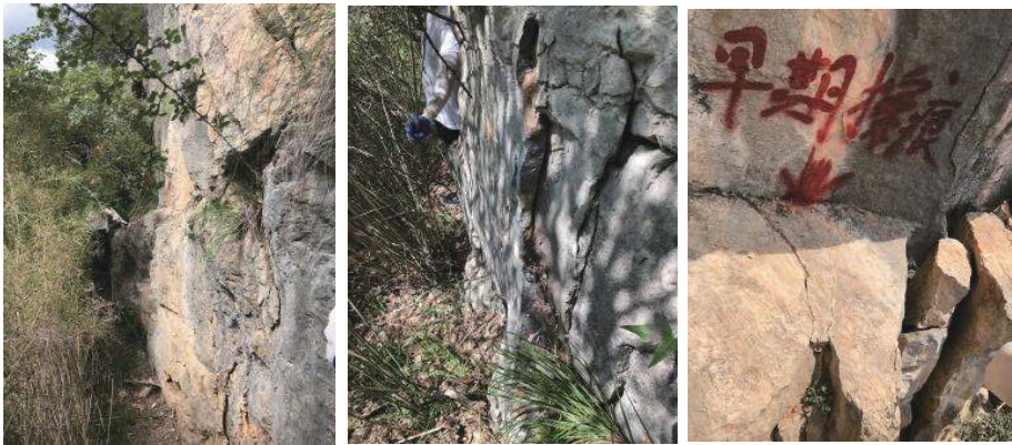
图 6 岸坡局部鼓胀、压裂及岸坡早期滑痕 Fig. 6 Local bulging, fracturing and early slippage of bank slope
