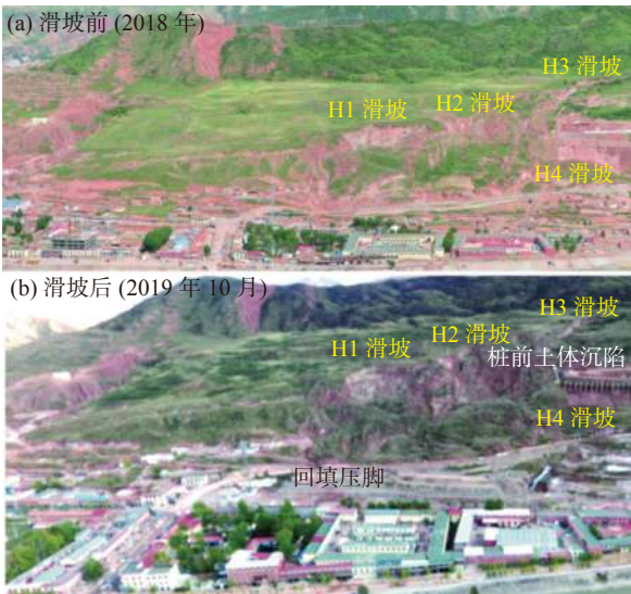
图 3 曲哇加萨滑坡发生前后对比 Fig. 3 Comparison before and after the occurrence of Quwajiasa landslide
