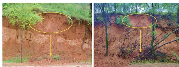
(a) G211-K504+85路侧坡顶滑塌 (b) G211-K506+190路侧坡顶滑塌
