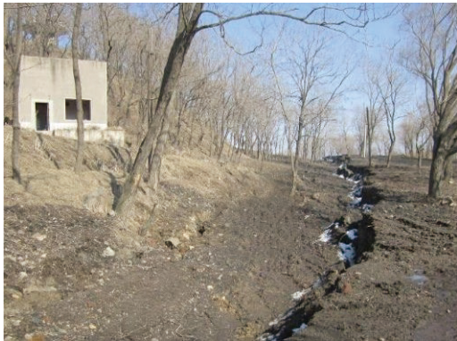
图 2 千台山滑坡裂缝 Fig. 2 Development of landslide cracks in Qiantai Mountain
