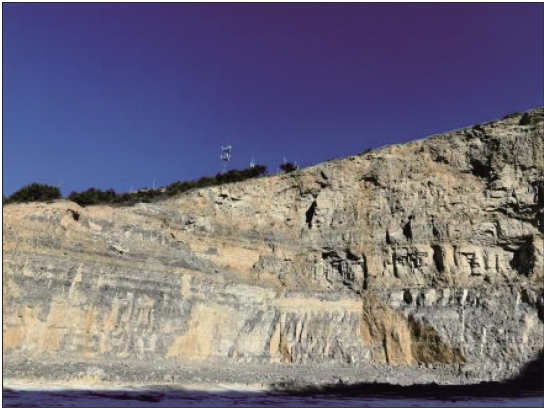
图1 研究区岩质边坡地形地貌特征 Fig.1 Topographic and geomorphological characteristics of the rock slope in the study area
