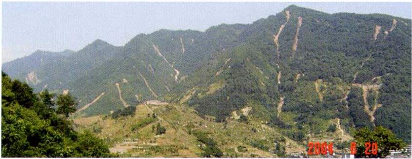
照片 1 宁陕县城北侧山坡坡面泥石流沟景观，照片上方山体均为 D_{2gnl} ，中下方为 \gamma_5^I 花岗岩，可见坡面流发育受 D_{2gnl} 岩层走向控制明显，镜头向 SE130^\circ Photo 1 Landscape of slope mudflow ravines on hill slopes north of the seat of Ningshaan County. The upper side of the photo is D_{2gnl} and the middle-lower side is granite ( \gamma_5^I ). The development of the slope mudflows are notably controlled by the strike of D_{2gnl} . looking toward S130^\circ E
