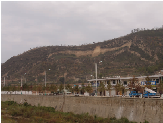
图2 虎头岭滑坡全貌 Fig. 2 Full view of the Hutoumao landslide
